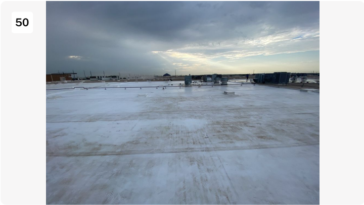
Project: cosmax building 1 Date: 7/21/2022, 7:46am Creator: Byron Johnson
