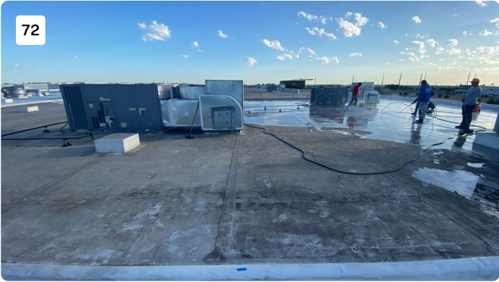
Project: cosmax building 1 Date: 7/25/2022, 7:49am Creator: Byron Johnson
