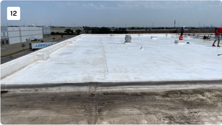
Project: cosmax building 1 Date: 7/18/2022, 11:38am Creator: Byron Johnson
