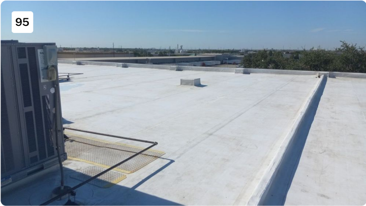
Project: cosmax building 1 Date: 7/27/2022, 9:44am Creator: Byron Johnson
