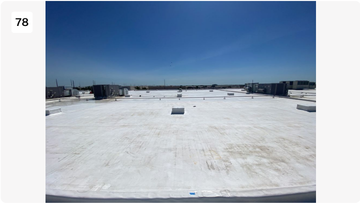
Project: cosmax building 1 Date: 7/26/2022, 11:36am Creator: Byron Johnson
