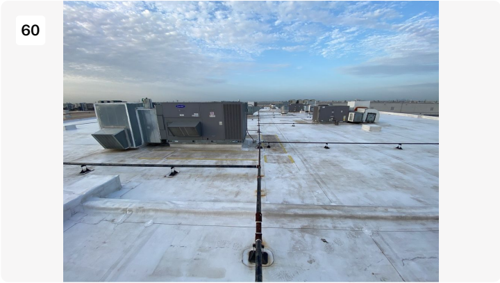
Project: cosmax building 1 Date: 7/22/2022, 7:17am Creator: Byron Johnson
