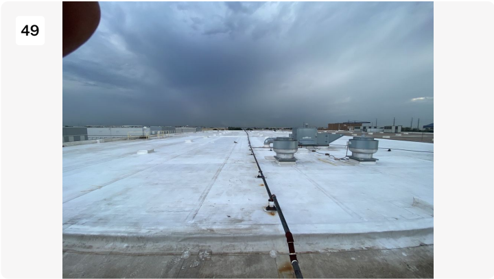
Project: cosmax building 1 Date: 7/21/2022, 7:45am Creator: Byron Johnson
