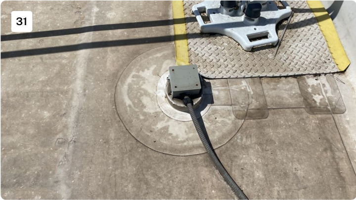
Project: cosmax building 1 Date: 7/19/2022, 11:10am Creator: Byron Johnson
