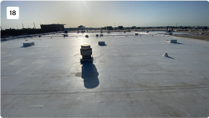
Project: cosmax building 1 Date: 7/19/2022, 8:15am Creator: Byron Johnson
