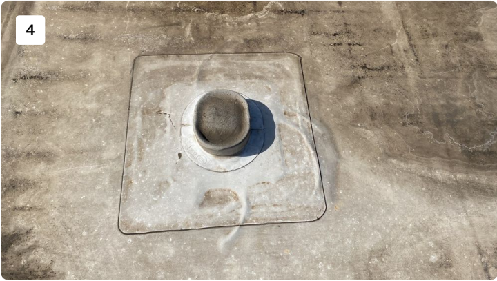
Project: cosmax building 1 Date: 7/18/2022, 9:38am Creator: Byron Johnson
