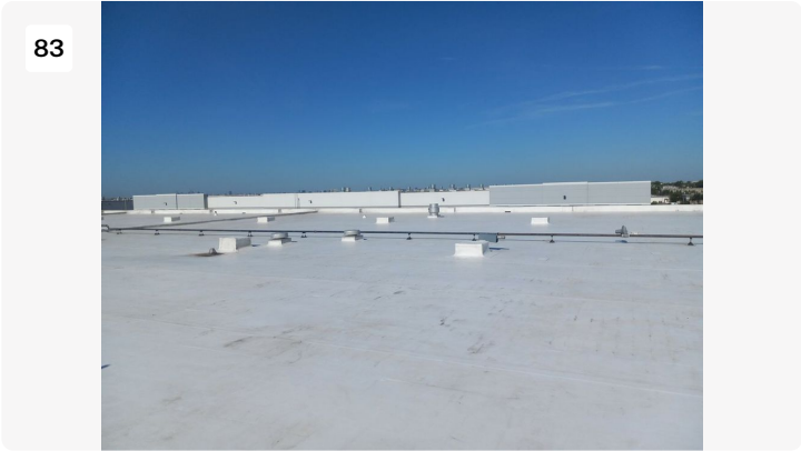
Project: cosmax building 1 Date: 7/27/2022, 9:33am Creator: Byron Johnson
