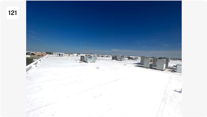
Project: cosmax building 1 Date: 8/1/2022, 12:29pm Creator: Craig Needham
