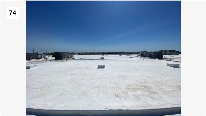
Project: cosmax building 1 Date: 7/26/2022, 11:33am Creator: Byron Johnson
