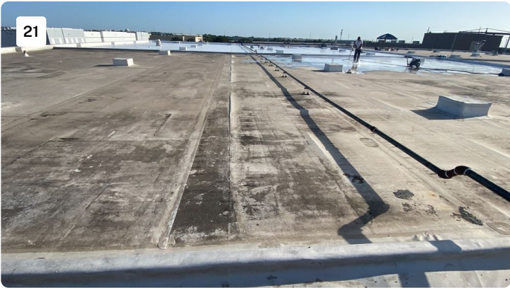
Project: cosmax building 1 Date: 7/19/2022, 8:18am Creator: Byron Johnson
