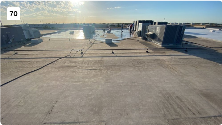
Project: cosmax building 1 Date: 7/25/2022, 7:42am Creator: Byron Johnson
