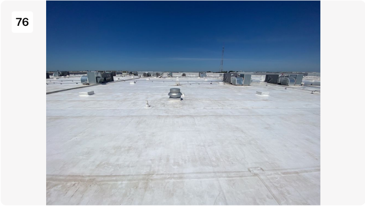
Project: cosmax building 1 Date: 7/26/2022, 11:35am Creator: Byron Johnson
