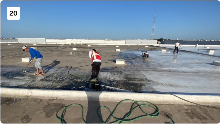
Project: cosmax building 1 Date: 7/19/2022, 8:17am Creator: Byron Johnson
