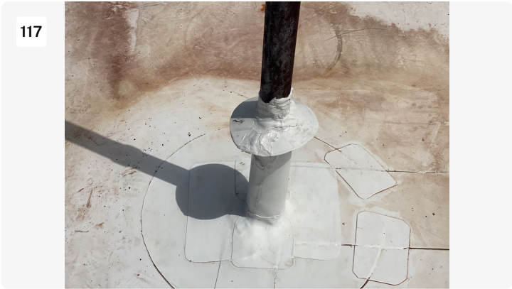
Project: cosmax building 1 Date: 8/1/2022, 12:00pm Creator: Byron Johnson
