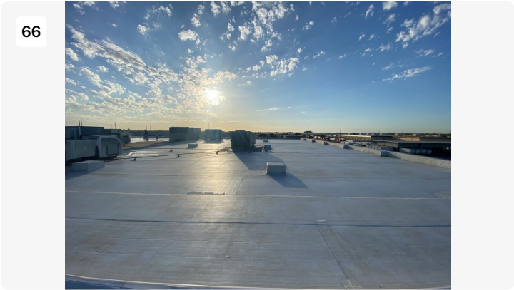
Project: cosmax building 1 Date: 7/25/2022, 7:38am Creator: Byron Johnson
