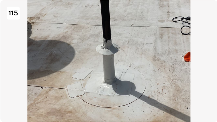
Project: cosmax building 1 Date: 8/1/2022, 11:59am Creator: Byron Johnson
