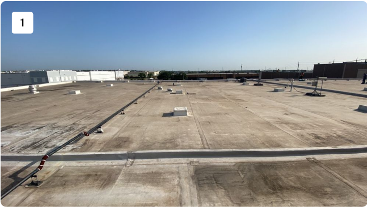
Project: cosmax building 1 Date: 7/18/2022, 8:52am Creator: Byron Johnson
