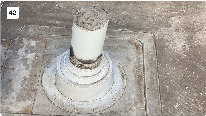
Project: cosmax building 1 Date: 7/20/2022, 9:48am Creator: Byron Johnson
