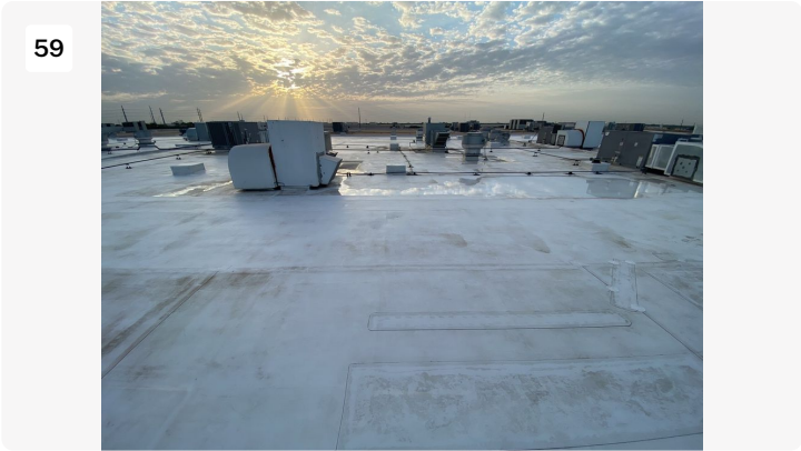
Project: cosmax building 1 Date: 7/22/2022, 7:16am Creator: Byron Johnson
