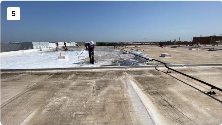
Project: cosmax building 1 Date: 7/18/2022, 10:36am Creator: Byron Johnson
