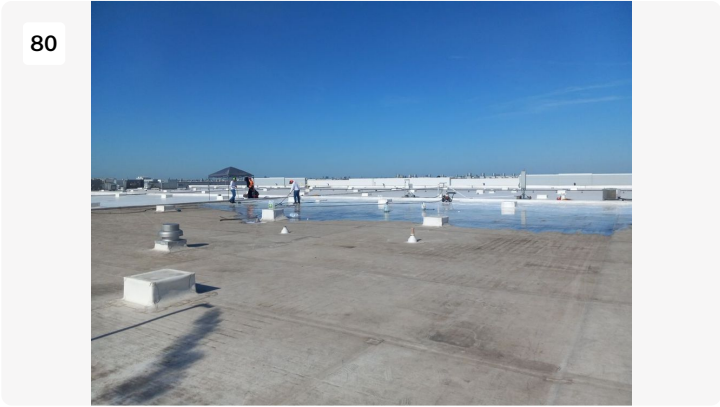
Project: cosmax building 1 Date: 7/27/2022, 9:32am Creator: Byron Johnson
