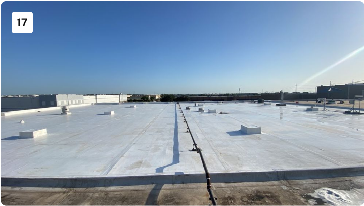
Project: cosmax building 1 Date: 7/19/2022, 8:14am Creator: Byron Johnson
