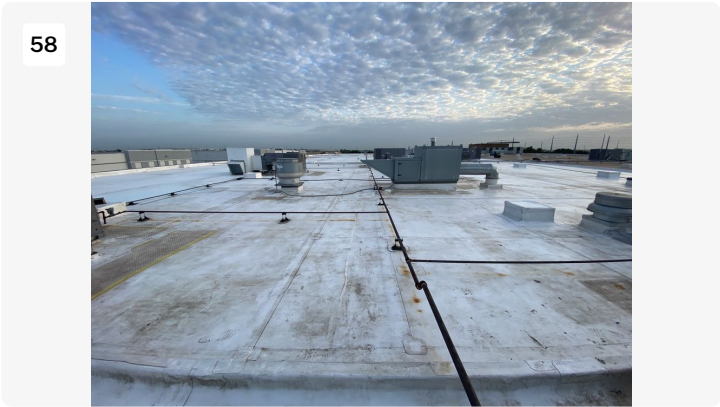
Project: cosmax building 1 Date: 7/22/2022, 7:15am Creator: Byron Johnson
