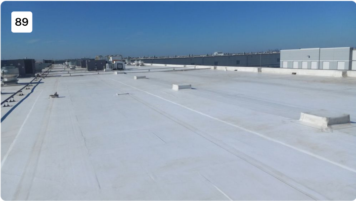
Project: cosmax building 1 Date: 7/27/2022, 9:41am Creator: Byron Johnson
