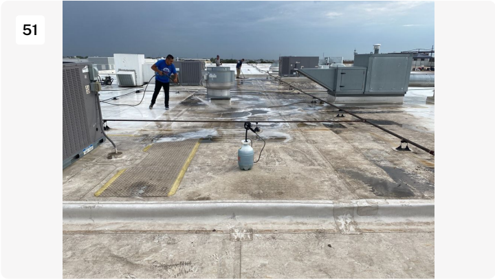
Project: cosmax building 1 Date: 7/21/2022, 9:29am Creator: Byron Johnson
