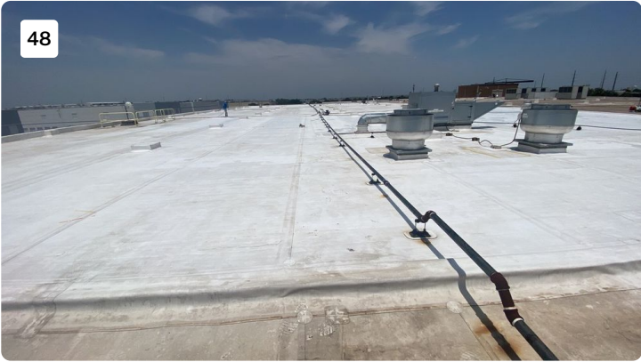
Project: cosmax building 1 Date: 7/20/2022, 1:41pm Creator: Byron Johnson
