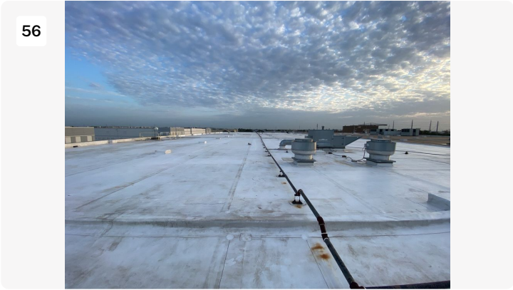
Project: cosmax building 1 Date: 7/22/2022, 7:11am Creator: Byron Johnson
