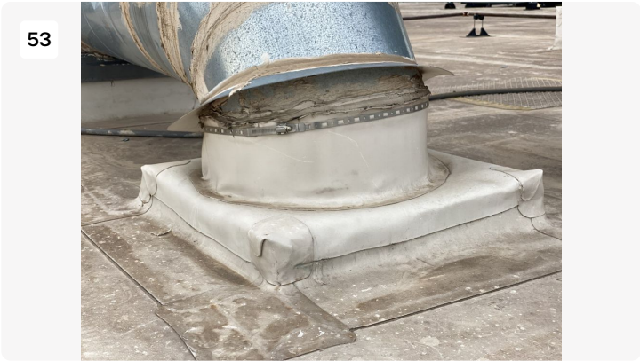
Project: cosmax building 1 Date: 7/21/2022, 10:10am Creator: Byron Johnson
