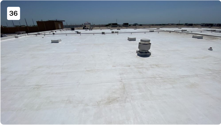
Project: cosmax building 1 Date: 7/19/2022, 11:57am Creator: Byron Johnson
