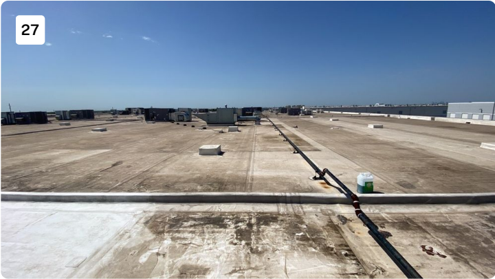
Project: cosmax building 1 Date: 7/19/2022, 11:08am Creator: Byron Johnson
