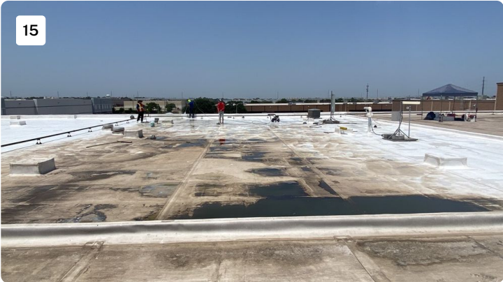
Project: cosmax building 1 Date: 7/18/2022, 2:25pm Creator: Byron Johnson
