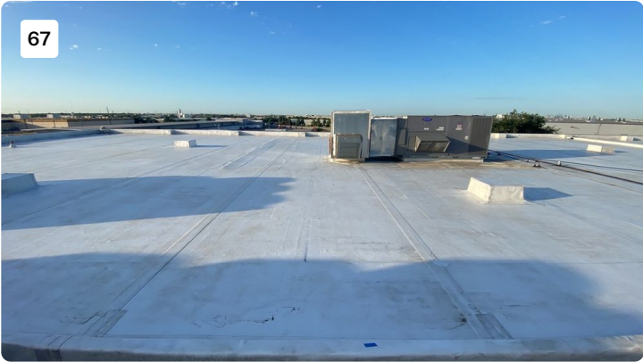
Project: cosmax building 1 Date: 7/25/2022, 7:39am Creator: Byron Johnson
