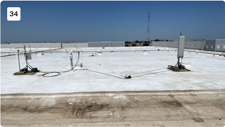
Project: cosmax building 1 Date: 7/19/2022, 11:54am Creator: Byron Johnson
