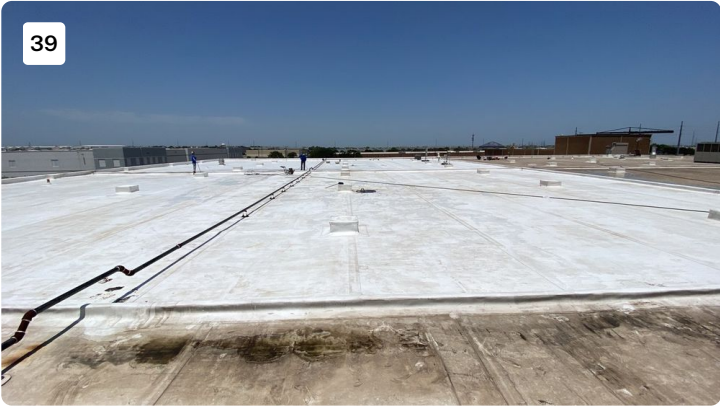
Project: cosmax building 1 Date: 7/19/2022, 1:45pm Creator: Byron Johnson
