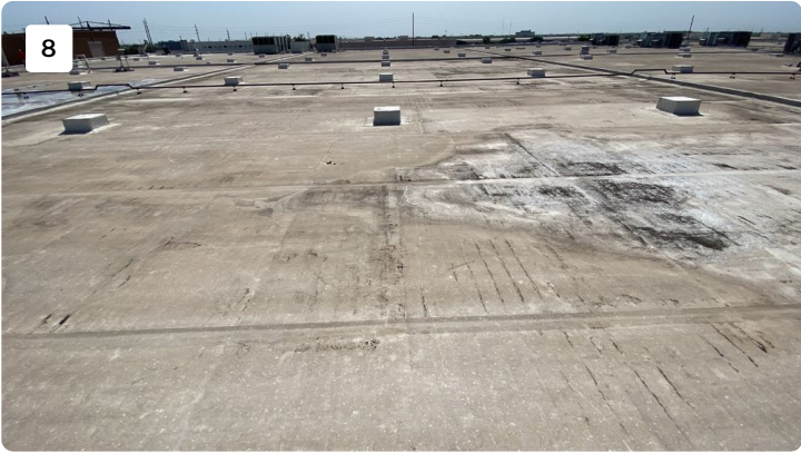
Project: cosmax building 1 Date: 7/18/2022, 10:39am Creator: Byron Johnson
