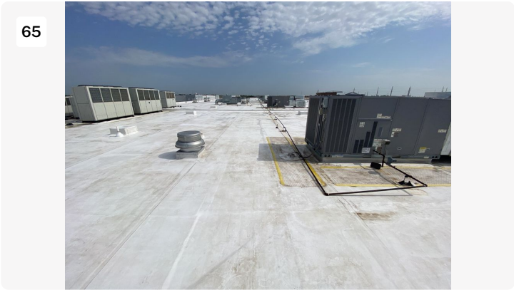
Project: cosmax building 1 Date: 7/22/2022, 10:19am Creator: Byron Johnson
