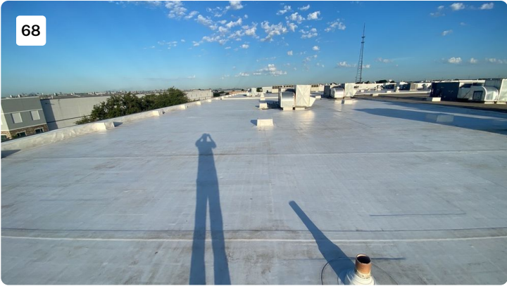
Project: cosmax building 1 Date: 7/25/2022, 7:40am Creator: Byron Johnson
