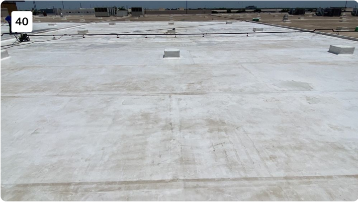
Project: cosmax building 1 Date: 7/19/2022, 1:46pm Creator: Byron Johnson
