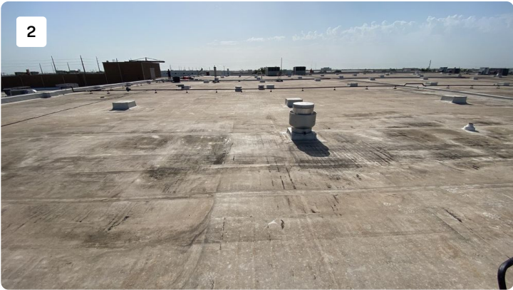
Project: cosmax building 1 Date: 7/18/2022, 9:37am Creator: Byron Johnson
