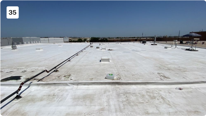
Project: cosmax building 1 Date: 7/19/2022, 11:55am Creator: Byron Johnson
