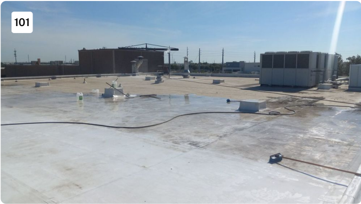
Project: cosmax building 1 Date: 7/27/2022, 9:47am Creator: Byron Johnson
