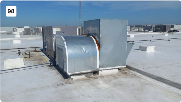
Project: cosmax building 1 Date: 7/27/2022, 9:45am Creator: Byron Johnson
