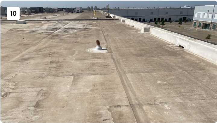
Project: cosmax building 1 Date: 7/18/2022, 10:40am Creator: Byron Johnson
