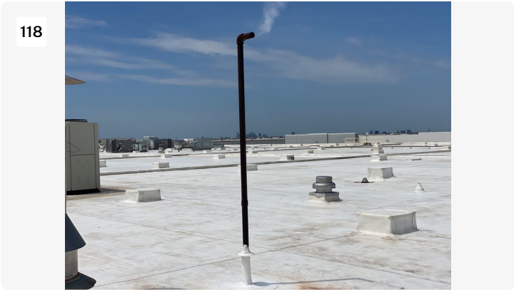
Project: cosmax building 1 Date: 8/1/2022, 12:03pm Creator: Byron Johnson
