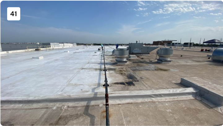
Project: cosmax building 1 Date: 7/20/2022, 9:47am Creator: Byron Johnson
