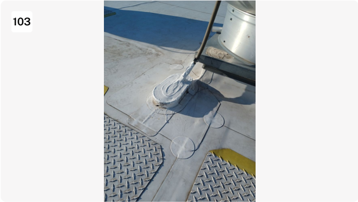
Project: cosmax building 1 Date: 7/29/2022, 9:38am Creator: Byron Johnson
