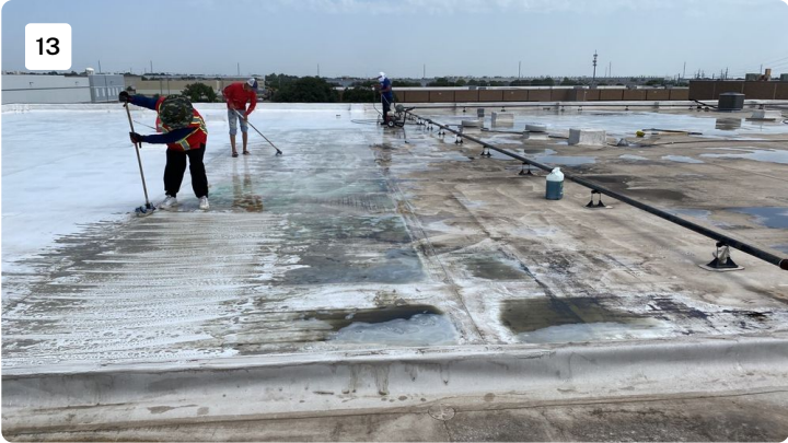
Project: cosmax building 1 Date: 7/18/2022, 11:38am Creator: Byron Johnson
