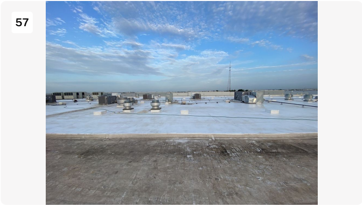
Project: cosmax building 1 Date: 7/22/2022, 7:14am Creator: Byron Johnson
