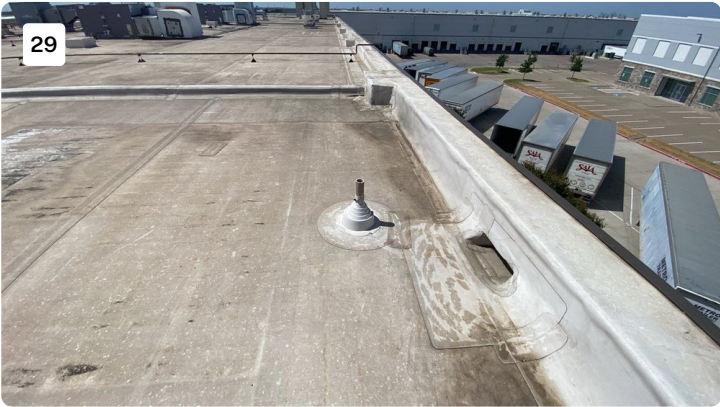
Project: cosmax building 1 Date: 7/19/2022, 11:09am Creator: Byron Johnson
