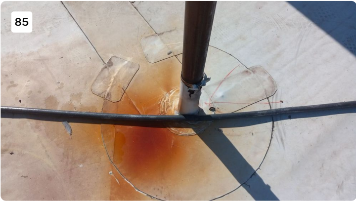
Project: cosmax building 1 Date: 7/27/2022, 9:38am Creator: Byron Johnson
