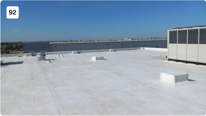
Project: cosmax building 1 Date: 7/27/2022, 9:43am Creator: Byron Johnson
