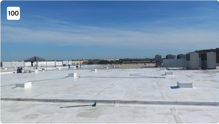
Project: cosmax building 1 Date: 7/27/2022, 9:46am Creator: Byron Johnson
