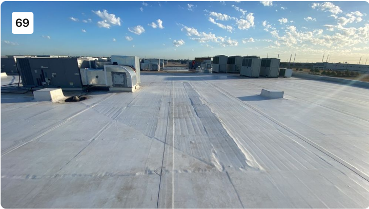
Project: cosmax building 1 Date: 7/25/2022, 7:41am Creator: Byron Johnson
