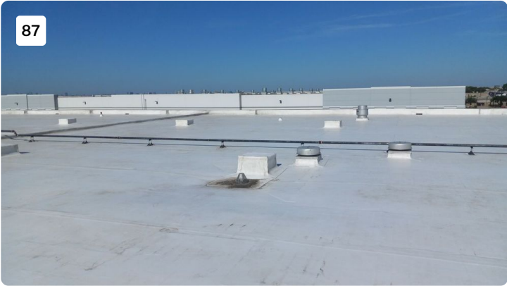
Project: cosmax building 1 Date: 7/27/2022, 9:39am Creator: Byron Johnson
