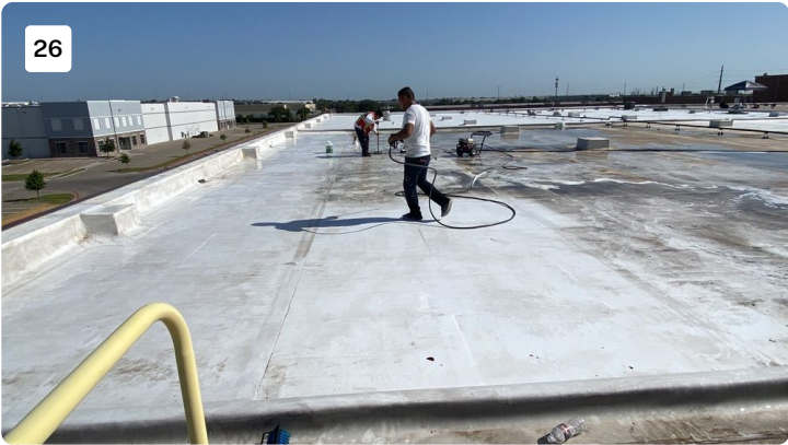
Project: cosmax building 1 Date: 7/19/2022, 9:51am Creator: Byron Johnson
