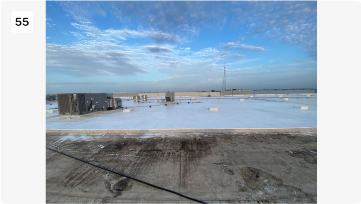
Project: cosmax building 1 Date: 7/22/2022, 7:09am Creator: Byron Johnson
