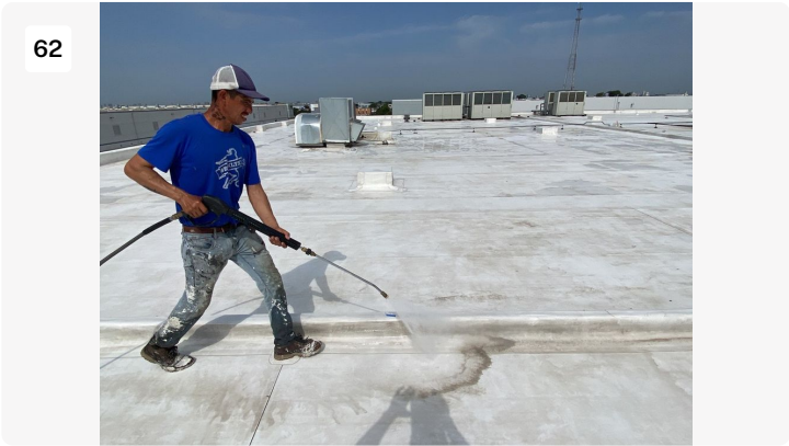
Project: cosmax building 1 Date: 7/22/2022, 10:18am Creator: Byron Johnson
