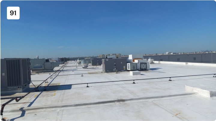
Project: cosmax building 1 Date: 7/27/2022, 9:42am Creator: Byron Johnson
