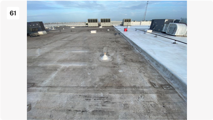
Project: cosmax building 1 Date: 7/22/2022, 7:21am Creator: Byron Johnson
