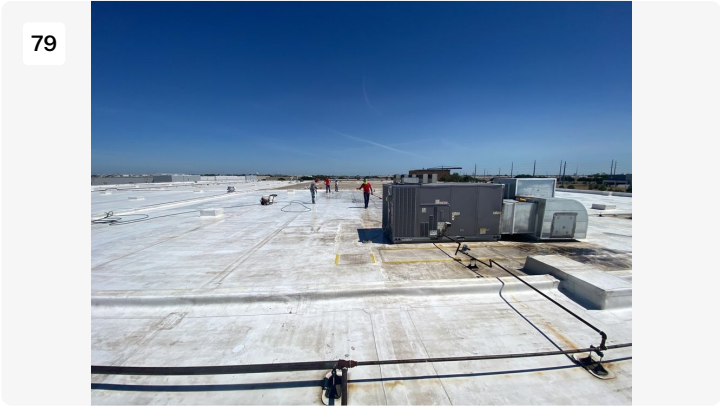
Project: cosmax building 1 Date: 7/26/2022, 11:37am Creator: Byron Johnson
