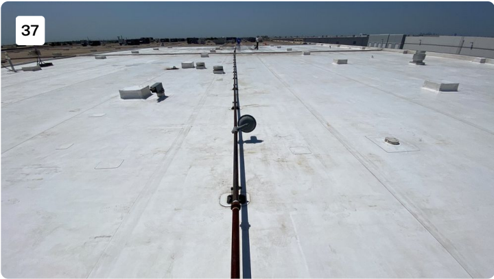
Project: cosmax building 1 Date: 7/19/2022, 12:01pm Creator: Byron Johnson
