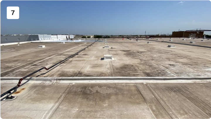
Project: cosmax building 1 Date: 7/18/2022, 10:38am Creator: Byron Johnson
