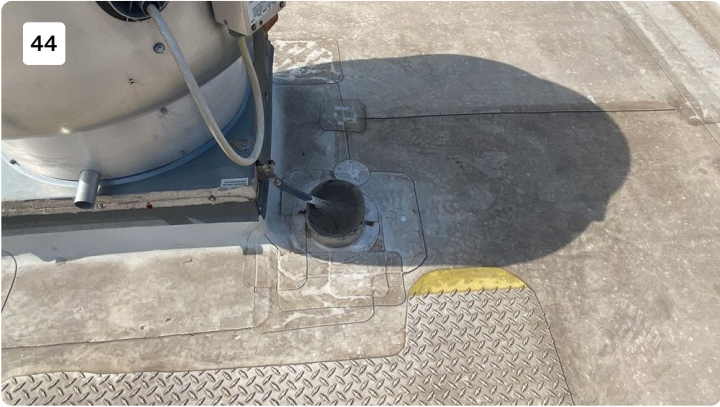
Project: cosmax building 1 Date: 7/20/2022, 9:53am Creator: Byron Johnson
