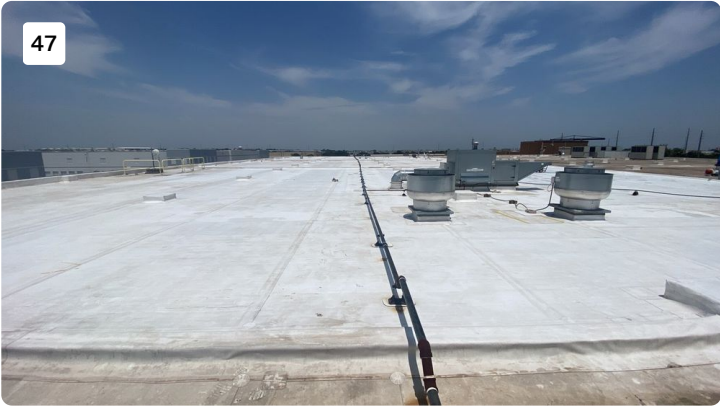
Project: cosmax building 1 Date: 7/20/2022, 1:30pm Creator: Byron Johnson
