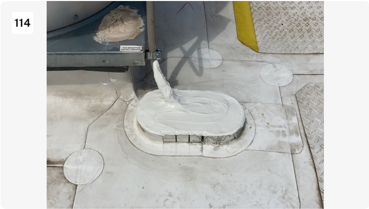
Project: cosmax building 1 Date: 8/1/2022, 11:56am Creator: Byron Johnson
