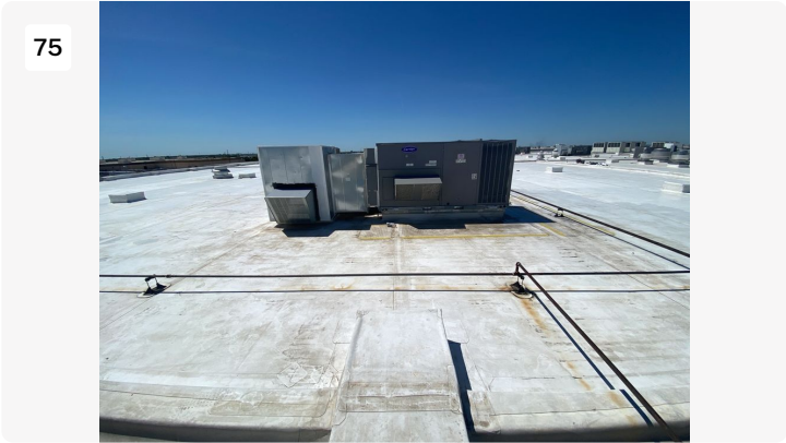
Project: cosmax building 1 Date: 7/26/2022, 11:34am Creator: Byron Johnson
