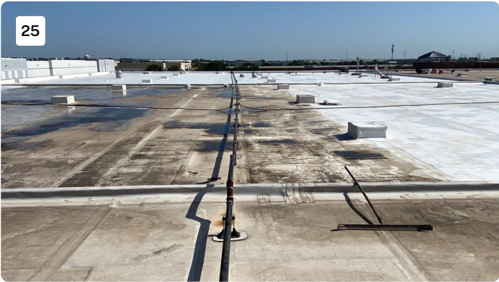
Project: cosmax building 1 Date: 7/19/2022, 9:50am Creator: Byron Johnson
