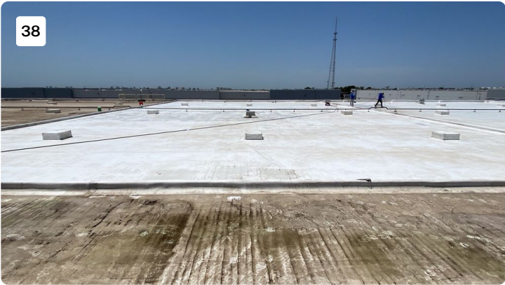
Project: cosmax building 1 Date: 7/19/2022, 1:42pm Creator: Byron Johnson
