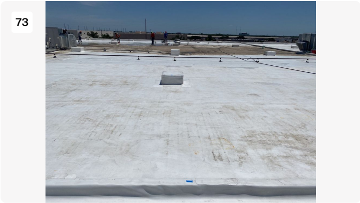
Project: cosmax building 1 Date: 7/25/2022, 1:08pm Creator: Byron Johnson
