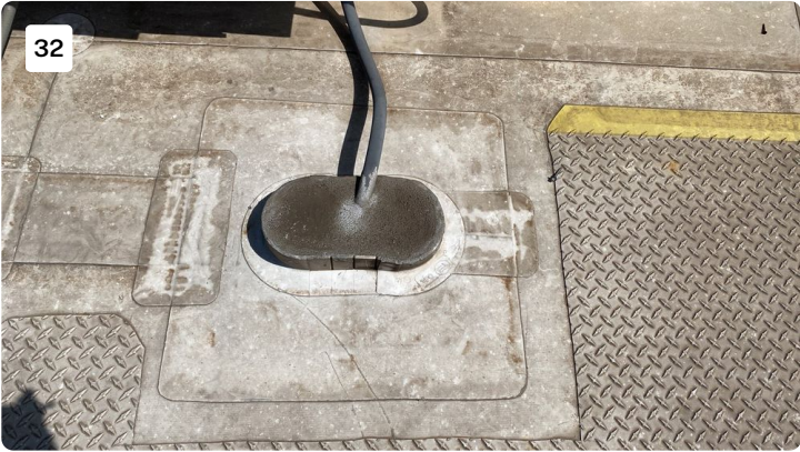
Project: cosmax building 1 Date: 7/19/2022, 11:11am Creator: Byron Johnson
